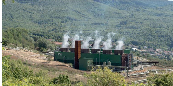
Bagnore 4 (Enel Green Power): 40 MW flash geothermal powerplant built in 2014
